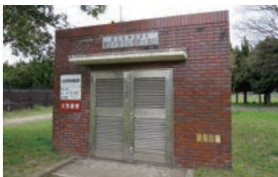
Emergency water supply tank
