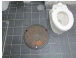
Manhole in a single room
